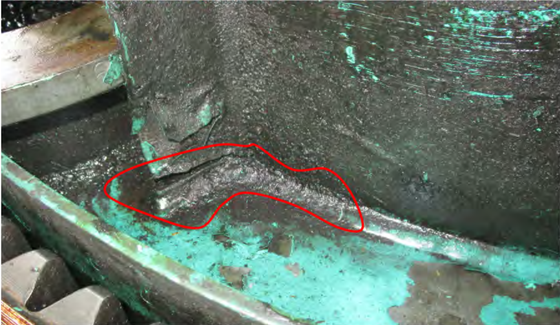
Image 3: Crack over the welding seam at an inner basket
