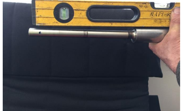
Removed bar showing bend
